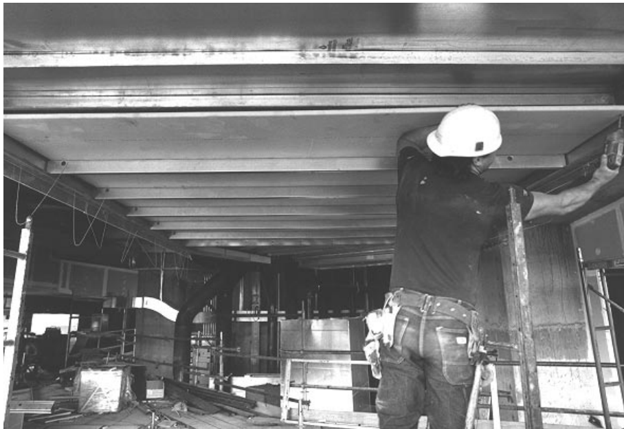
Fig. 6. Typical horizontal shaft wall installation under ductwork starts with USG Steel C-H Stud framing installed below ductwork, with SHEETROCK brand Gypsum Liner Panels installed between the studs (a). This is followed by application of triple-layer 1/2-in. SHEETROCK brand Gypsum Panels, FIRECODE C Core (b). Large size of ducts enclosed in USG Cavity Shaft Wall System is apparent (c).
