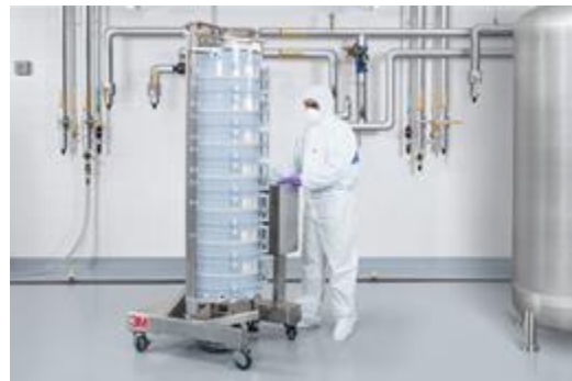
Figure 4f. 3M™ Zeta Plus™ Encapsulated System Filter Capsules (Production capsules) installed in 3M™ Encapsulated System Holders
