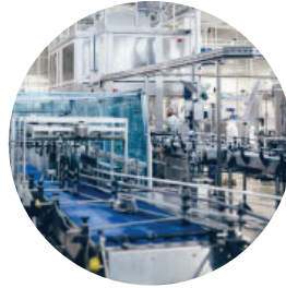
Industrial Water Systems
