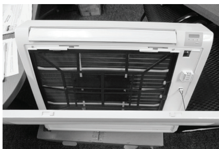
Figure 7. MFMA Typical Filter Removal
