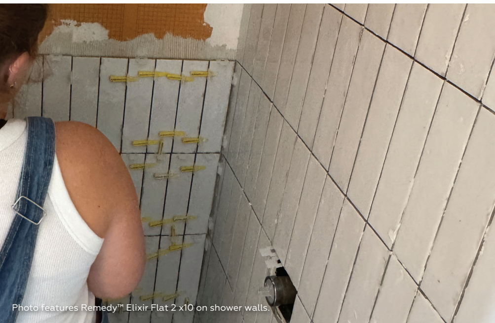
Photo features Remedy™ Elixir Flat 2 x10 on backsplash.
