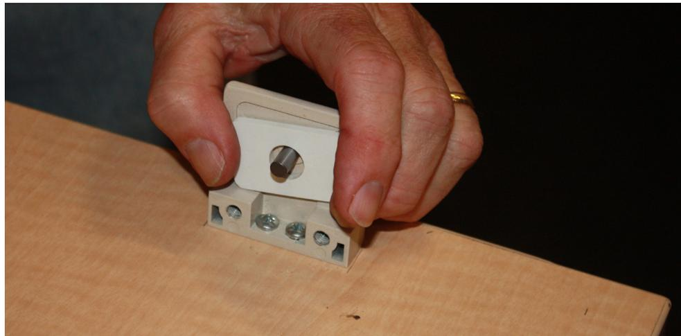
9. Take the mullion and line up the holes with the pegs on either PGHM. Then place the mullion onto the PGHM pegs.
