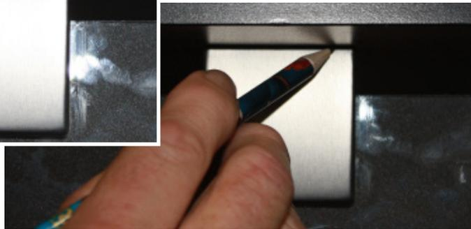
2. Worksurface/Panel does not have the holes drilled upon arrival. To start, put PGHM on mullion and then hold in place on the work surface.
