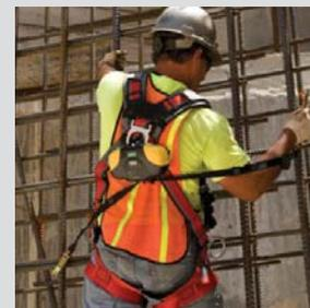
*Free-hanging from back D-ring, with lines extended downward for connection at or below the back D-ring.*
