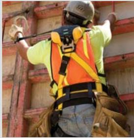
*Tightly secured to the harness using Velcro straps, with lines extended upward for overhead connection applications.*
