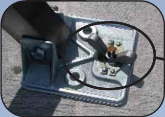
Two possible methods of securing stanchion feet to concrete
