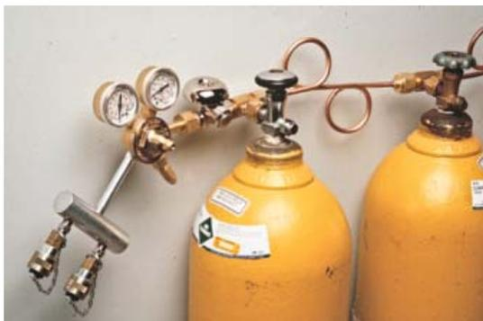
*Air cylinders connected by tee blocks and pigtails, equipped with Audi-Larm Audible Alarm and air cylinder pressure regulator.*
