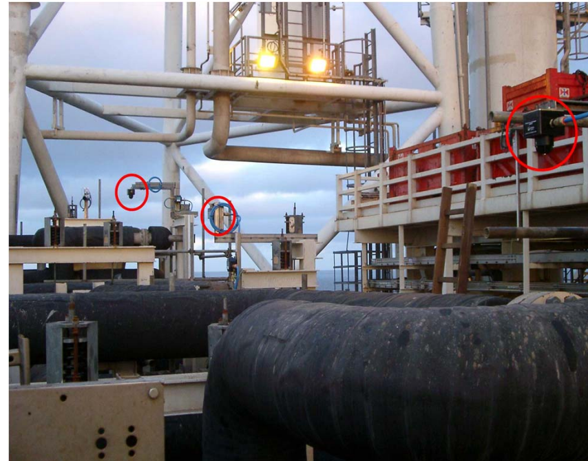
7 out of 9 Ultrasonic detectors installed on a Hess weather deck in the North Sea.
