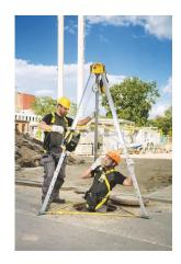
Confined space entry and retrieval equipment may be necessary to facilitate both entry into and exit from confined spaces. Proper fall protection systems for workers comprise anchorage (e.g. tripod), full-body harness, connecting devices (e.g. retractable lifeline, winch / rescue unit).
