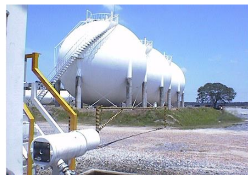
Figure 14: OPGD monitoring at boundary of LPG storage tank farm
