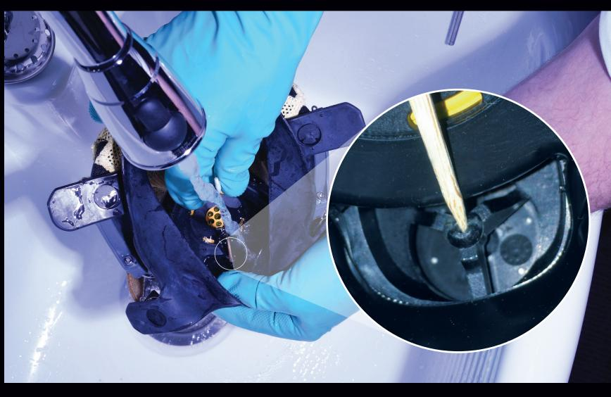
5. Flush and manually operate the exhalation valve assembly by depressing the stem with a blunt, dull object. Be careful not to damage any rubber components on the facepiece.
