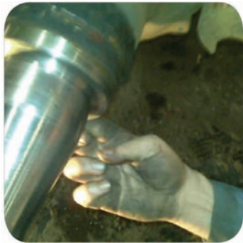
Visually check underside as well
